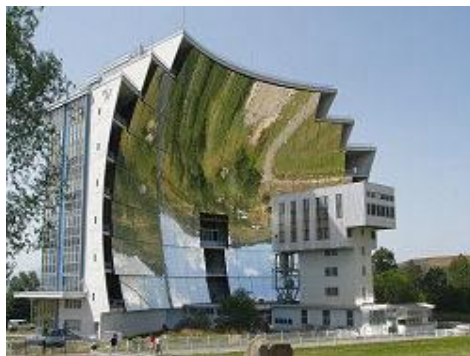
Fig: The Solar Furnace of Odeillo; the parabolic shape of the giant solar collector is evident here.
