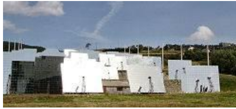
Fig: The array of mirrors is controlled by a computer and turn with the sun.
