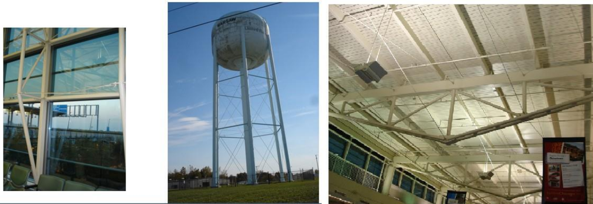
Tie Rods in Structures
